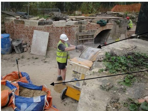
Lime being placed in the mixer; note the mask, safety glasses and gloves. Note also the high-viz, the eyewash is hidden from view
